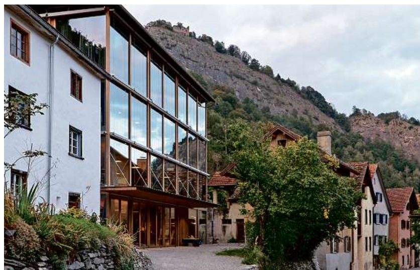
... das neue Atelier Zumthor in Haldenstein ...
