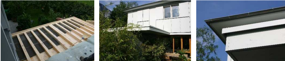
Anbau Velounterstand, Ems
